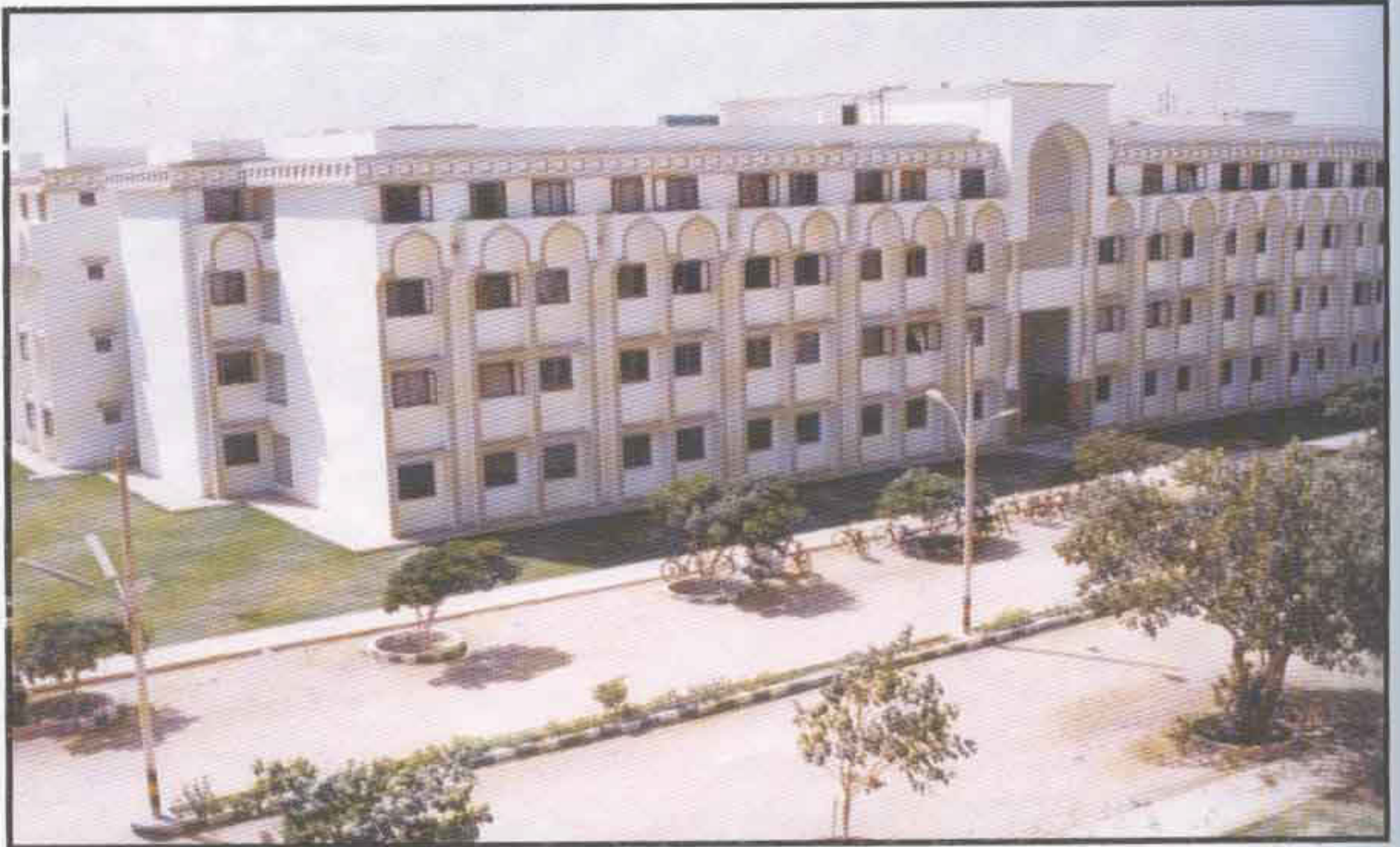
A view of the Student Hostel from south west. The building has been artistically landscaped with beautiful greenery on all four sides which generates a sense of peace for its residents.
